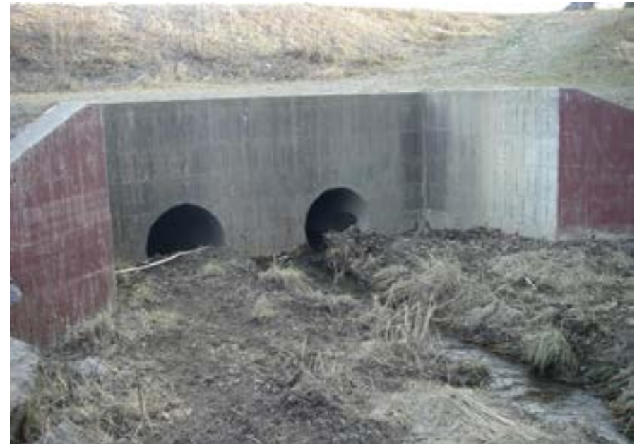
Fairview Avenue culverts. Source: Bill Spencer.
