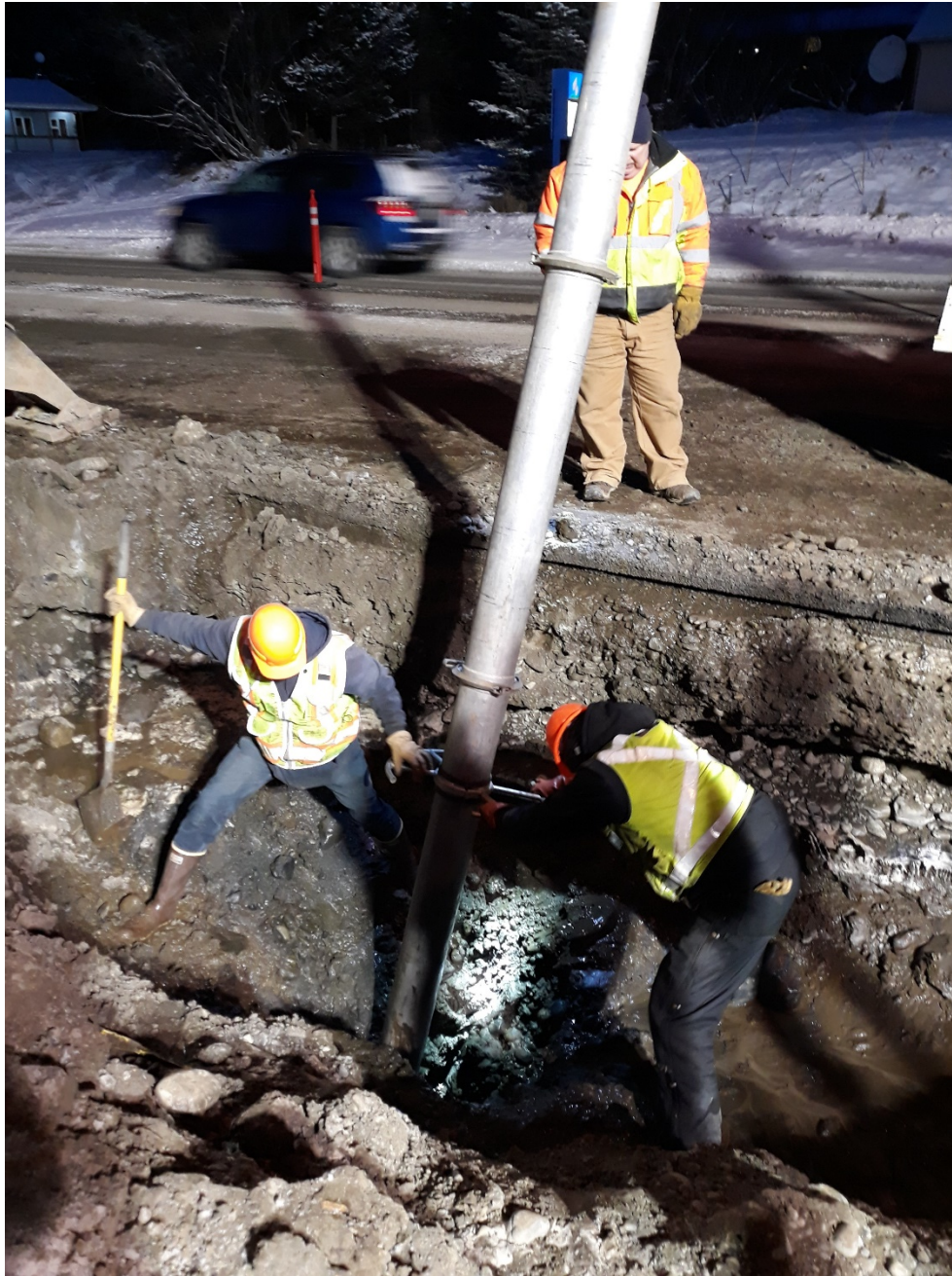
The photo above shows Paul Raymond (at street level), Jason Hanenberger, and Mike Szocinski working on the Pioneer Avenue water main break.
