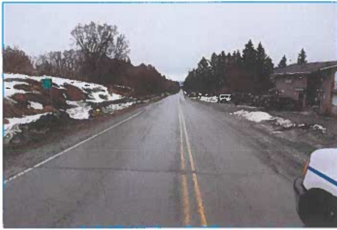
Fairview Ave looking east
