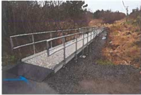
ADA ramp on Poopdeck Extension Trail
