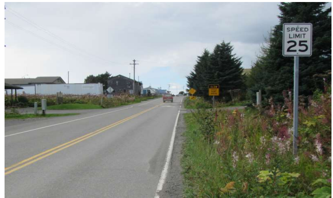
Figure 5- Speed Hump and Signage on Bunnell Avenue
