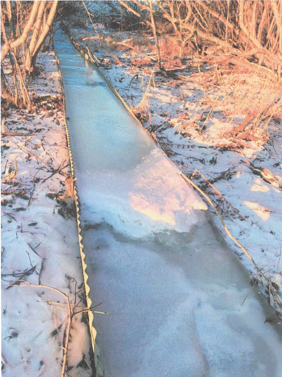
Photo 1. Iced full and breached half-culvert stormwater discharge alongside the Metz subject property.
