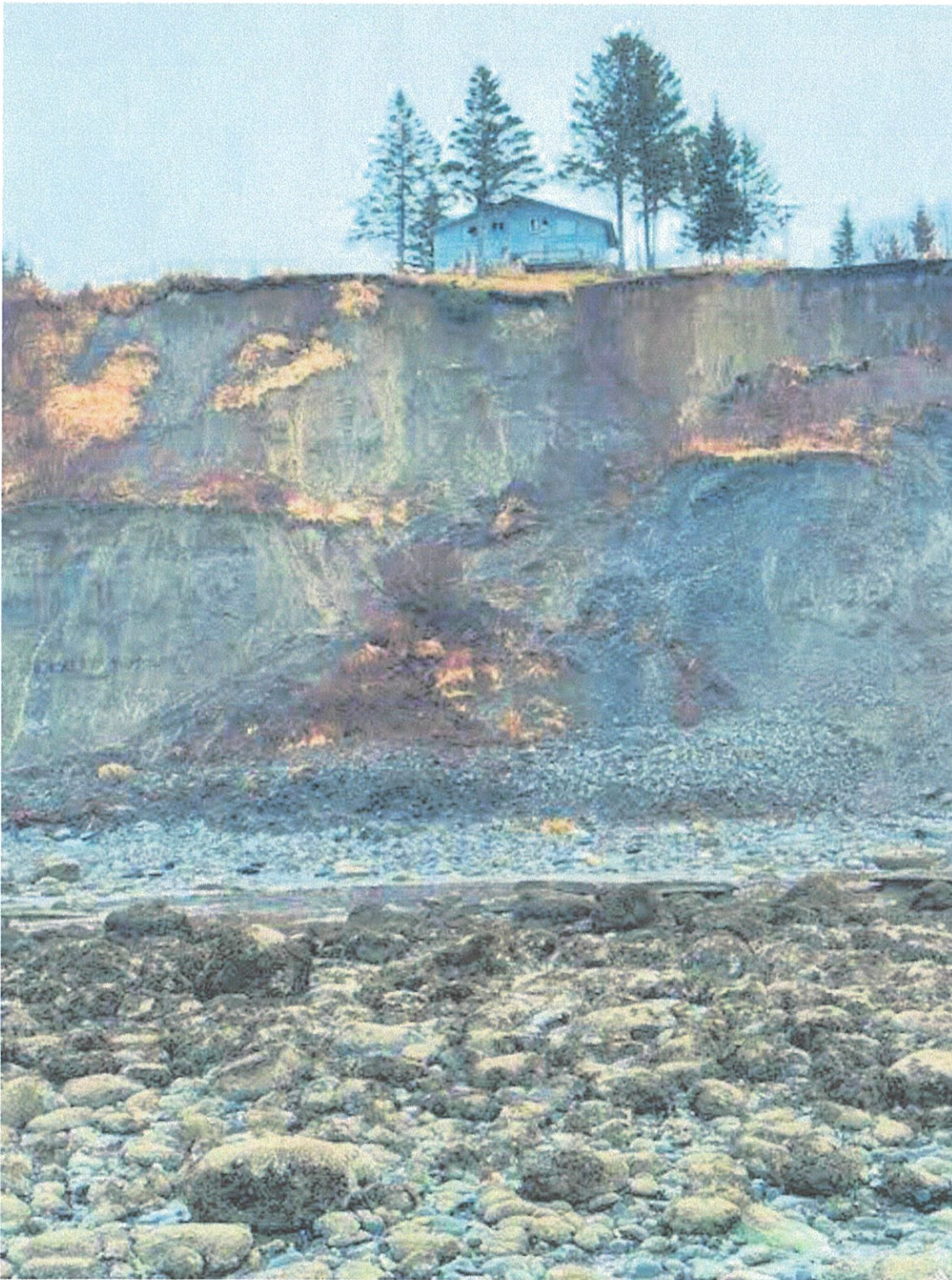
Photo 7. View of the entire sloughed bench and its importance to the stability of the Metz home.
