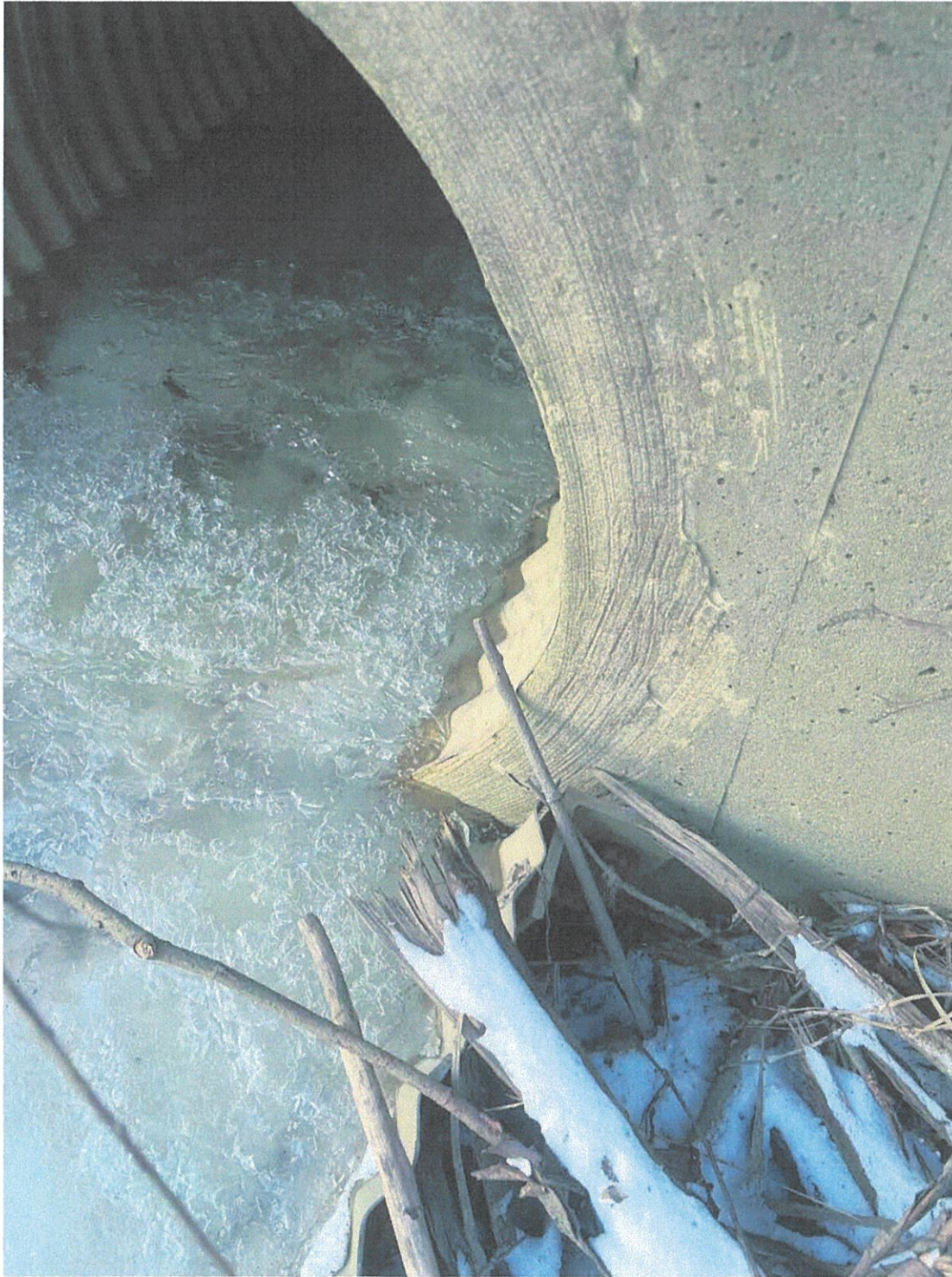
Photo 3. Outlet headwall leakage presumably begins the streamflow component underneath the half-culvert system
