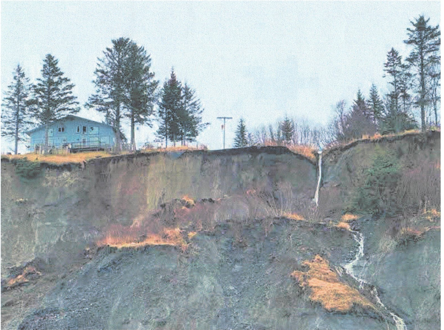
Photo 6. Stormwater discharge shown adjacent to the Metz property. Note that the recent slumping as a result of material saturation has diverted a significant amount of the stormwater to the left along the top of the sloughed material in front of the Metz home, creating an imminent mass wasting situation for the sloughed material – noting that this is all that is left supporting the Metz bluff.
