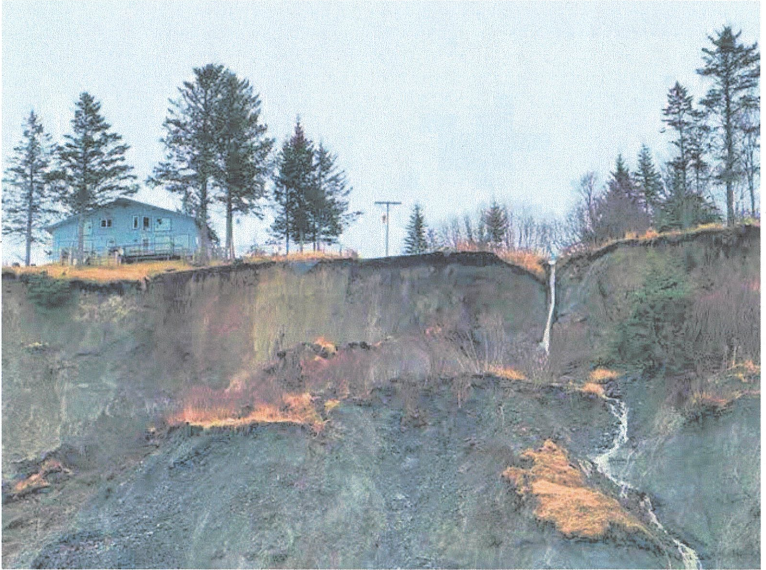
Photo 4. Stormwater discharge from the previous bluff-side half-culvert system now dumping into sloughed material and flowing both in front of the Metz house shown as well as to the right of the sloughed material.
