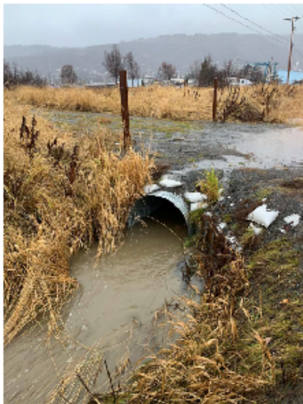
Photo 1. Turbid water about to be discharged from Kachemak Bay as direct runoff from the industrial areas and boatyard, showing visible particulate and flooding of the Kachemak Bay drainage ditch, illustrating the small outflow that is usually here, October 30th, 2022
