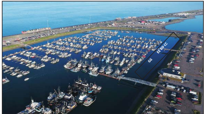
System 4 ramps to be replaced next.
