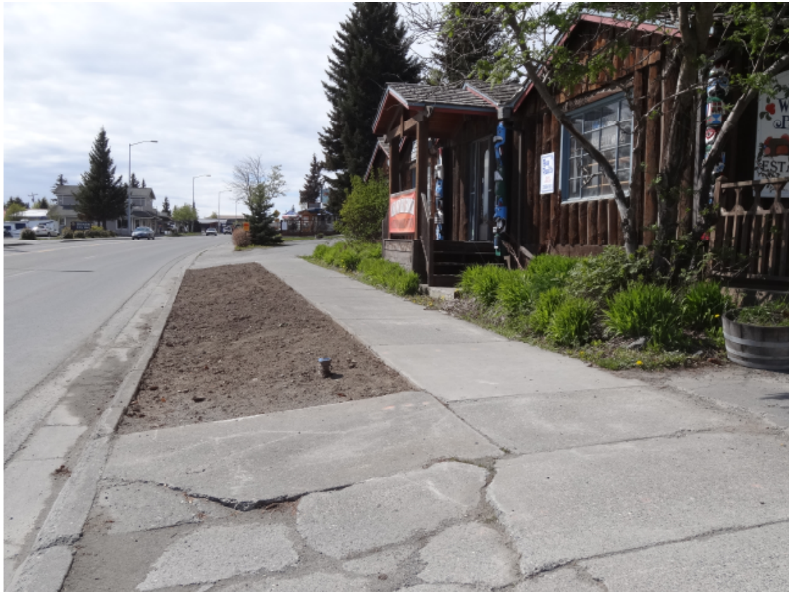
Pic of Wildberry Products After sod removal
