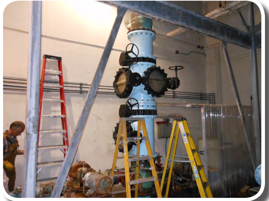
Installing the UV system at Trail Lakes Hatchery.
