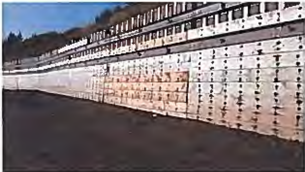
Repair made to panel section
