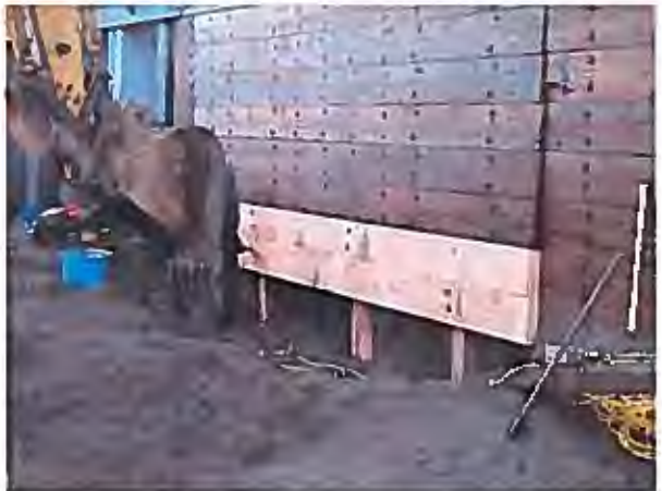
Lower wall repair - 2011
