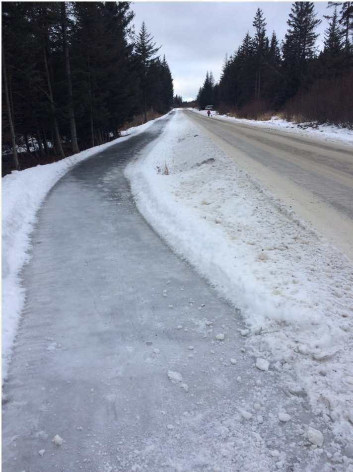
Spruceview Avenue Separated Sidewalk Unsanded
