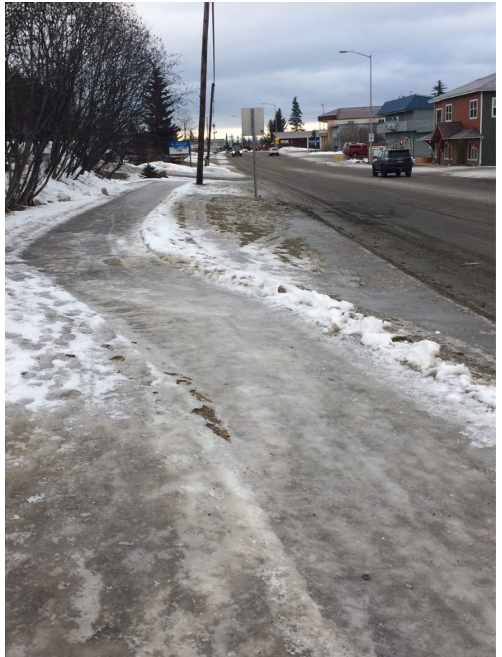
Pioneer Avenue Separated Sidewalk Unsanded
