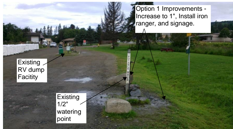
Existing Public Works RV Dump Site
