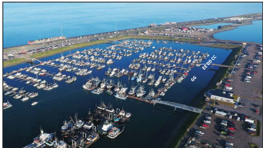
System 4 ramps to be replaced next.
