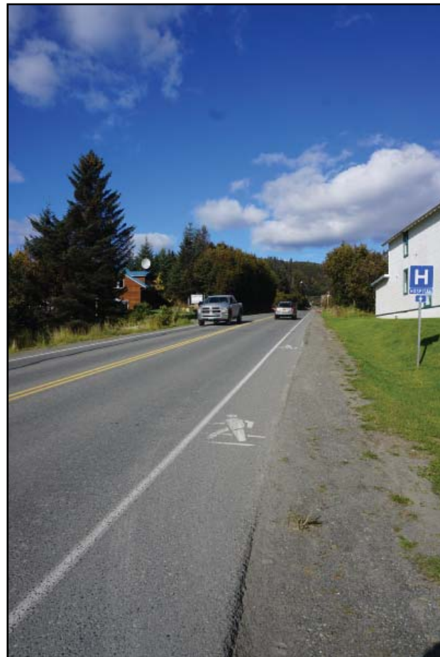
Pedestrian safety along Main Street, one of Homer’s primary north-south roads, would benefit from a sidewalk facility.
