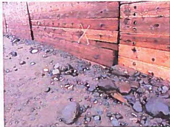
Lower wall repair - 2017
