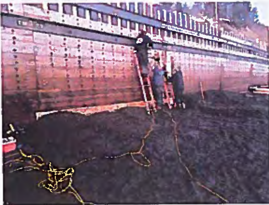
Repair made to panel
