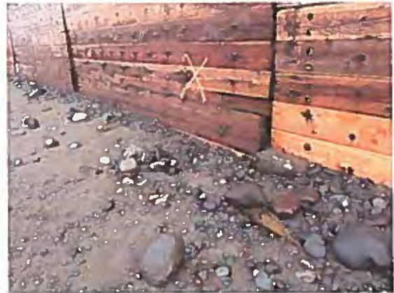
Lower wall repair - 2017
