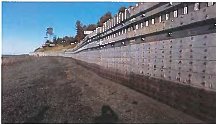
Sand/gravel summer build up protects toe of wall from erosion
