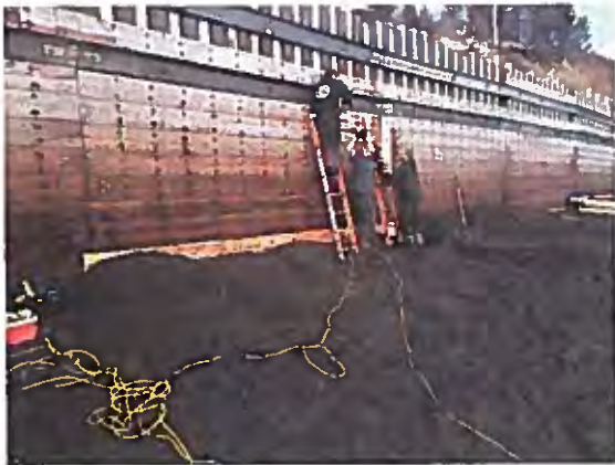
Repair made to panel
