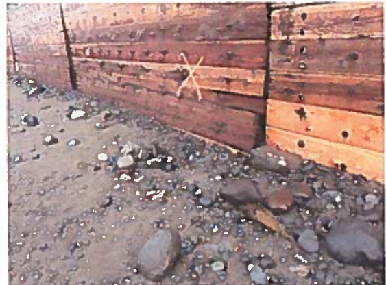
Lower wall repair - 2017
