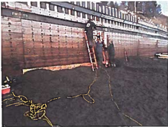
Repair made to panel
