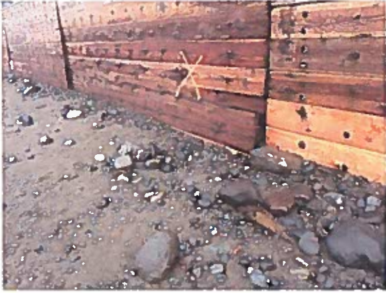
Lower wall repair - 2017
