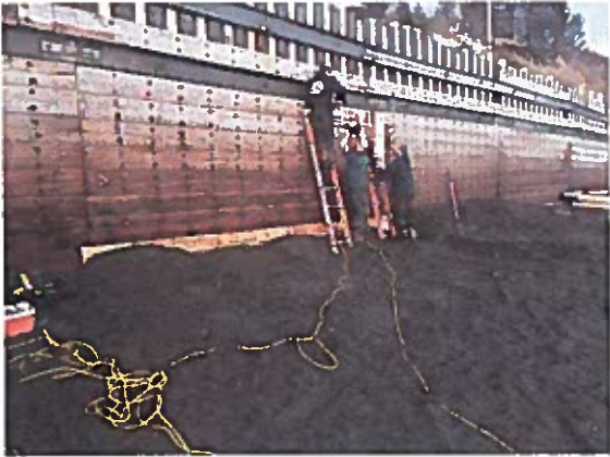
Repair made to panel
