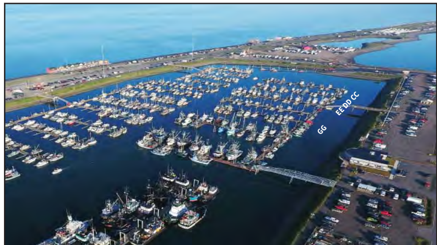
System 4 ramps to be replaced next.
