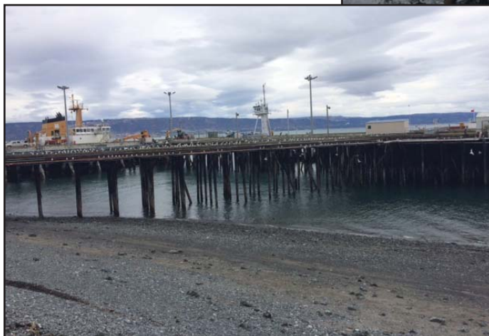
The former Main Dock in Homer's Port & Harbor is over fifty years old, defunct and deteriorated to the point that it is a hazard and a liability.
