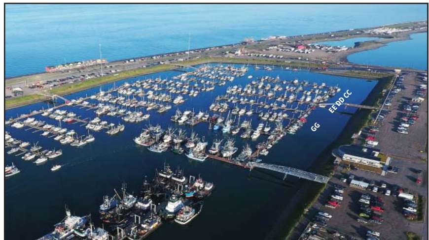
System 4 ramps to be replaced next.
