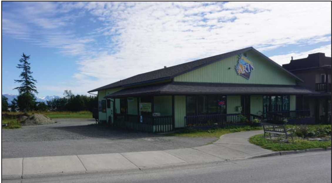
HCOA is designing a major addition to its current facility: the Mary Epperson Performing Arts Center, a black-box style theater located behind the HCOA offices in the grassy field behind the gravel pile in the photo above.
