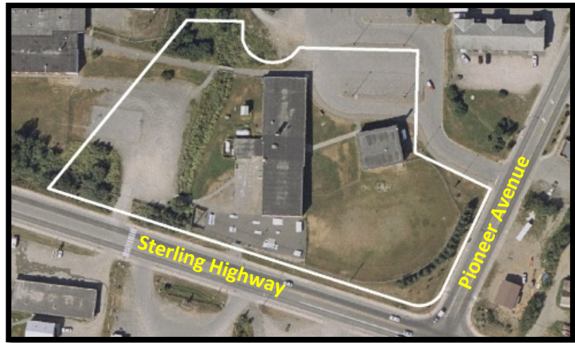
2003 photograph of the HERC property. HERC-1 (on left) is the focus of this report. HERC-2 (on right), is only discussed in terms of demolition costs.
