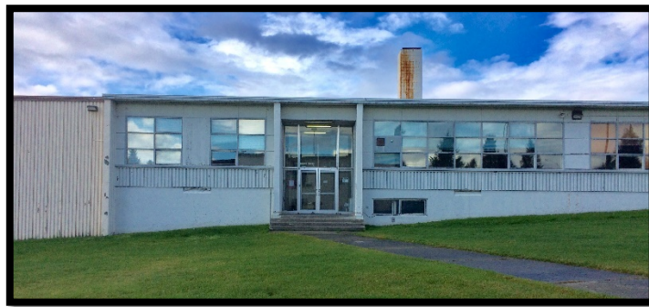
HERC-1 Upper Level Entrance
