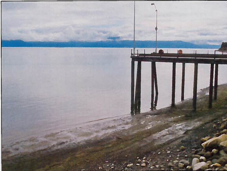
Looking SE to the subject tidelands lot beginning near the end of the dock and extending into Kachemak Bay 167'+/-. The photo was taken about 1 hour after a high tide of 14.9' with all of the tidelands mostly under water.
