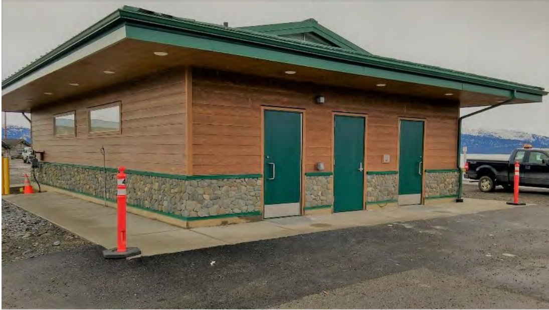
New Ramp 2 Restrooms
