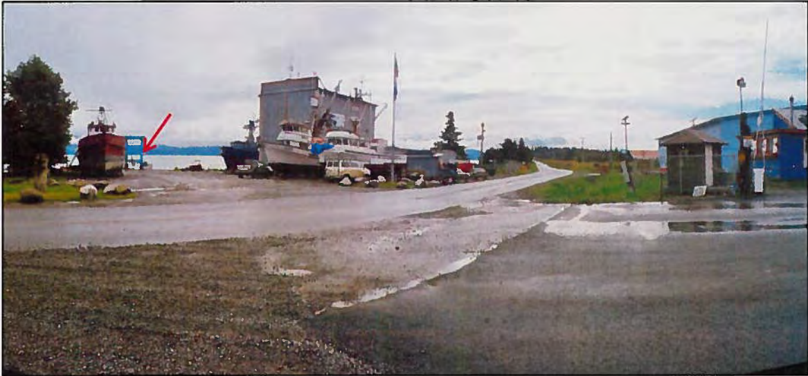
Looking SE over Kachemak Dr. to the subject uplands at left. Driveway in foreground at right is to the Northern Enterprises Boat Yard. The dock on the uplands/tideland lots is partially visible at arrow.
