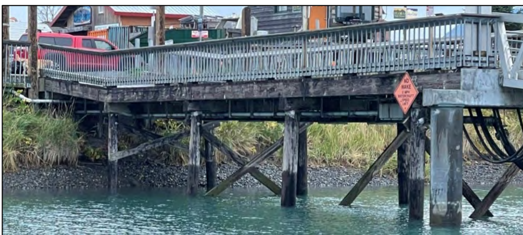
Figure 2.4: Ramp 2 timber pile supported trestle.
