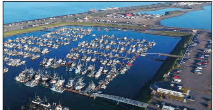
System 4 floats to be replaced.
