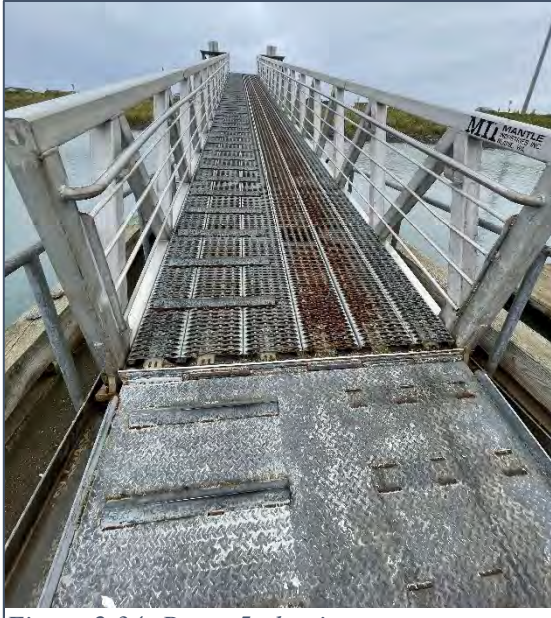
Figure 2.34: Ramp 5 aluminum gangway w steel floor grating.
