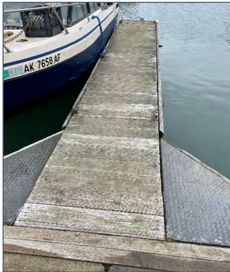
Figure 2.41: concrete stall float with decking attached over the top.
