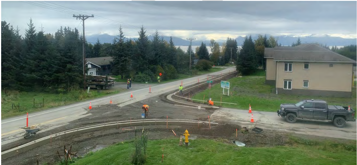
Figure 1 - Crews working on the Main Street Sidewalk completed in fall 2022
