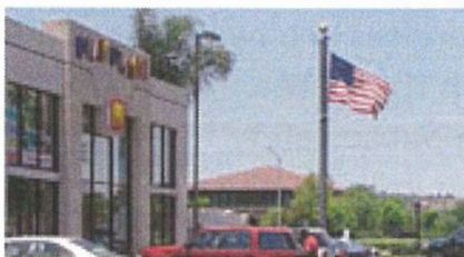
☐ Figure 6 Tower Disguised as Flag Pole
