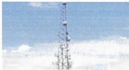
⊕ Figure 2 Typical Lattice Tower
