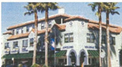
☐ Figure 5 Tower Disguised as Chimney
