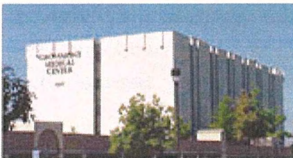
▣ Figure 3 Representative Facade Mounted Antennae
