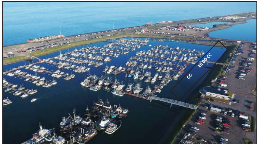
System 4 ramps to be replaced next.
