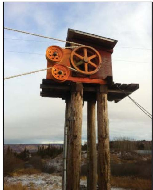
Ohlson Mountain Rope Tow's top station, which supports the engine, bullwheel and weight of the rope in motion, is in need of foundation repair.
