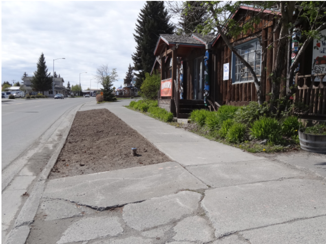
Pic of Wildberry Products After sod removal
