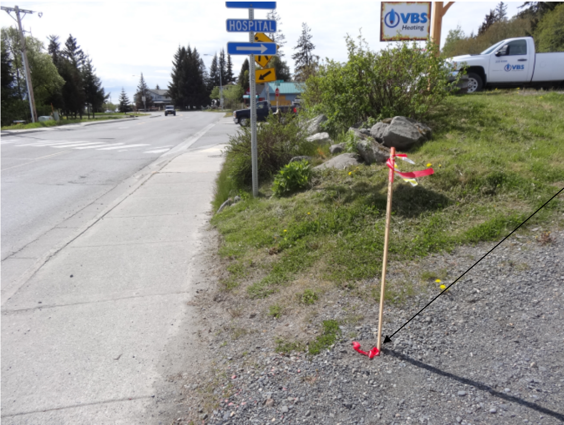
View looking west on north side of Pioneer at VBS Heating
