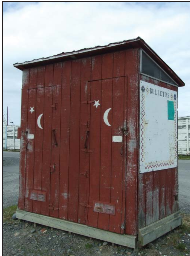
Ramp 8 sees heavy use from crews of large vessels moored in System 5. Since this outhouse was removed in 2015, crews walk 1.5 blocks to use the nearest restroom facility.
