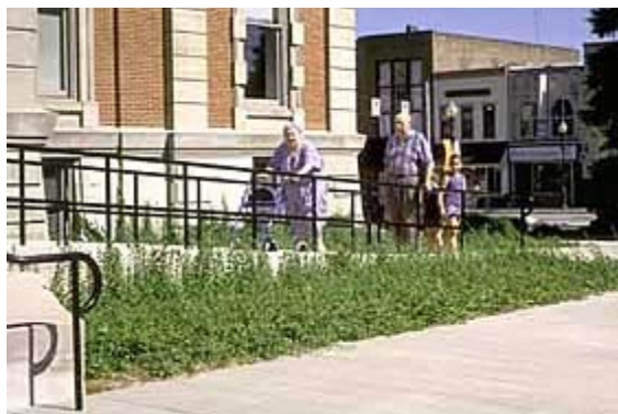
A historic town building added a ramp, walkway, and modified an entrance to provide access
