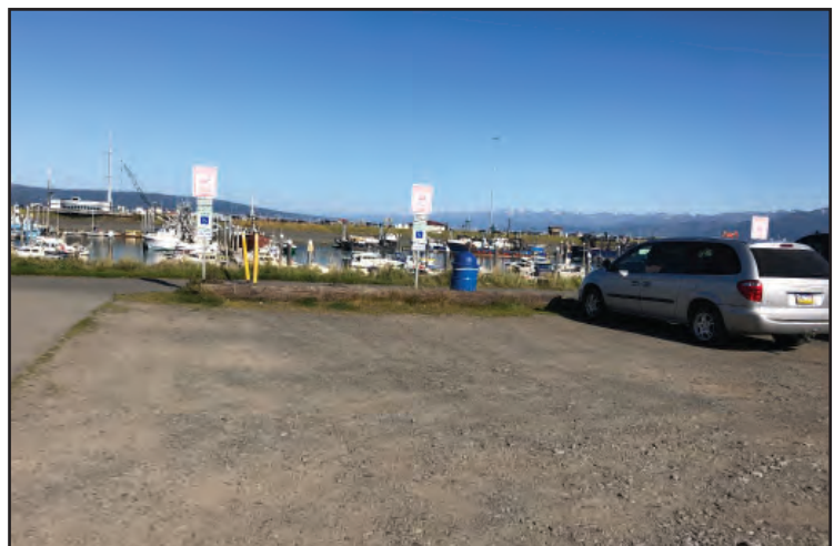
Accessible parking spaces at Ramp 4 in the Port & Harbor provide an example of where spaces need to be paved and a path of travel provided to the sidewalk.
