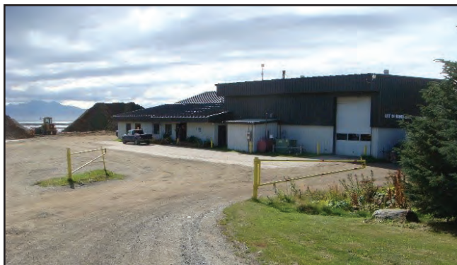
City of Homer existing Public Works facility.
