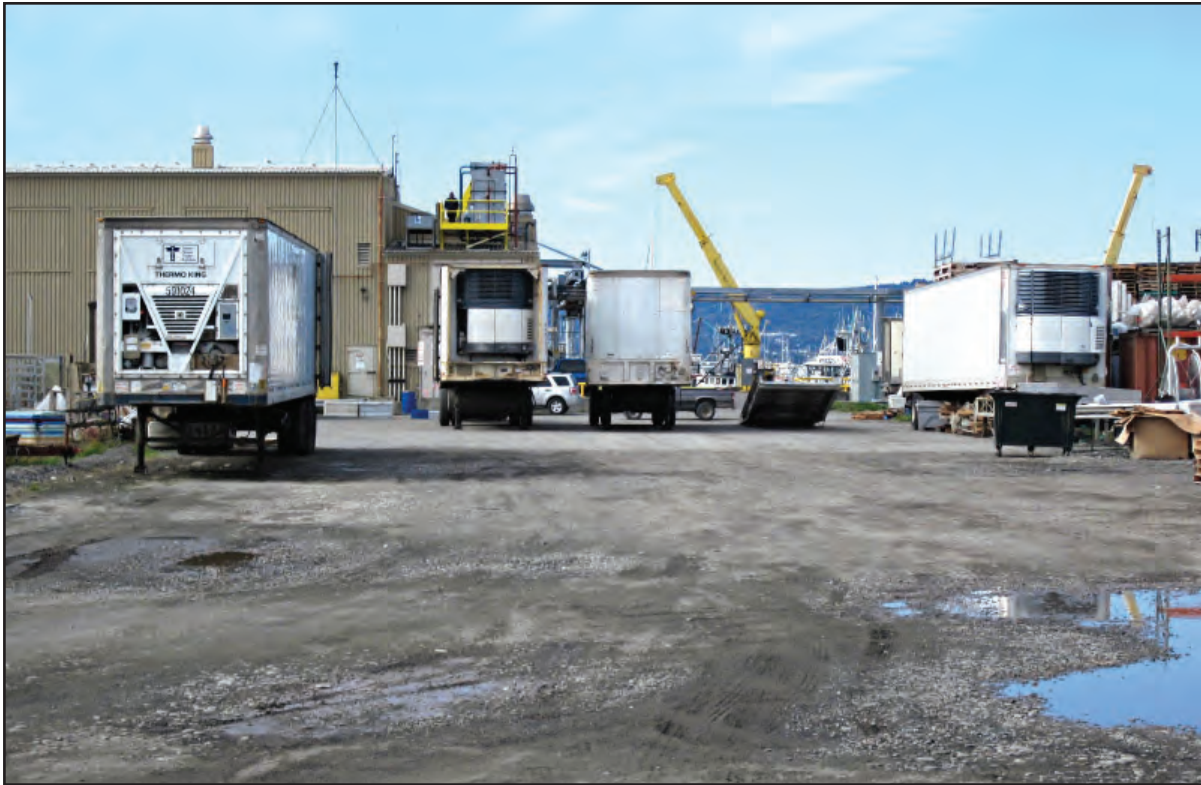
Currently at the Fish Dock, fish buyers have to contend with a muddy lot and lack of a loading dock to facilitate the transfer of fish to trucks.
