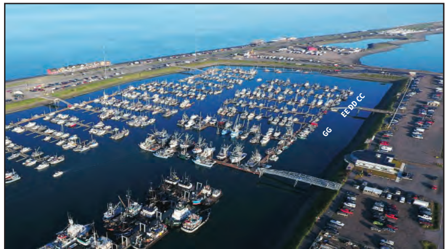
System 4 ramps to be replaced next.
