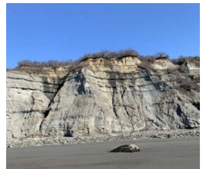
Seepage can be seen flowing from the bluff face.
