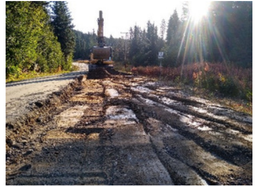
Road surface removed on Sprucewood Drive.
