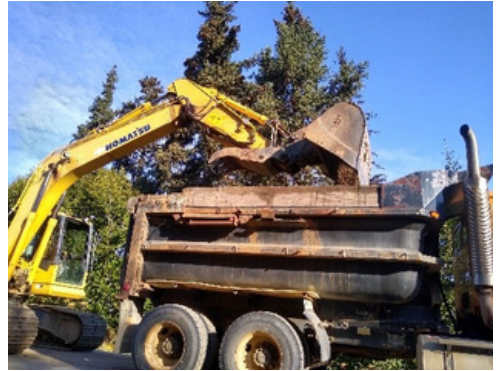
Unusable material loaded into dump truck for haul off.
