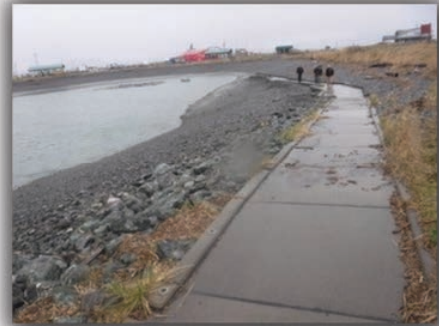
ADA sidewalk/ramp at the Nick Dudiak Fishing Hole.
