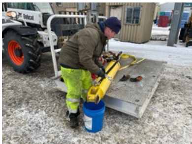
Replacement cylinder on the platform ready for installation.
