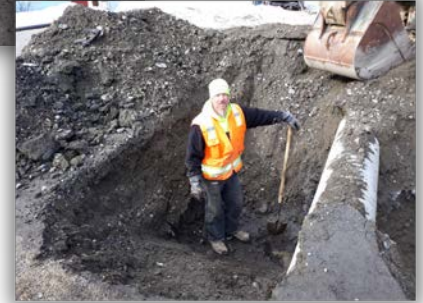
Below: James Trissell, W/S crew in the trench.
