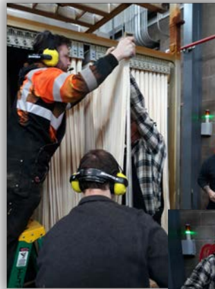
Left: Sean Love taking down a rack of water filter membranes to examine.
