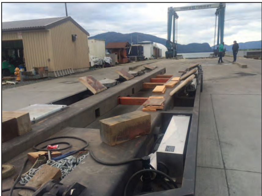
An example of a sling lift and adjacent repair yard area.
