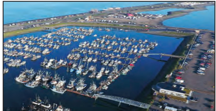
System 4 floats to be replaced.
