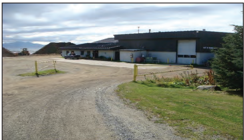
City of Homer existing Public Works facility.
