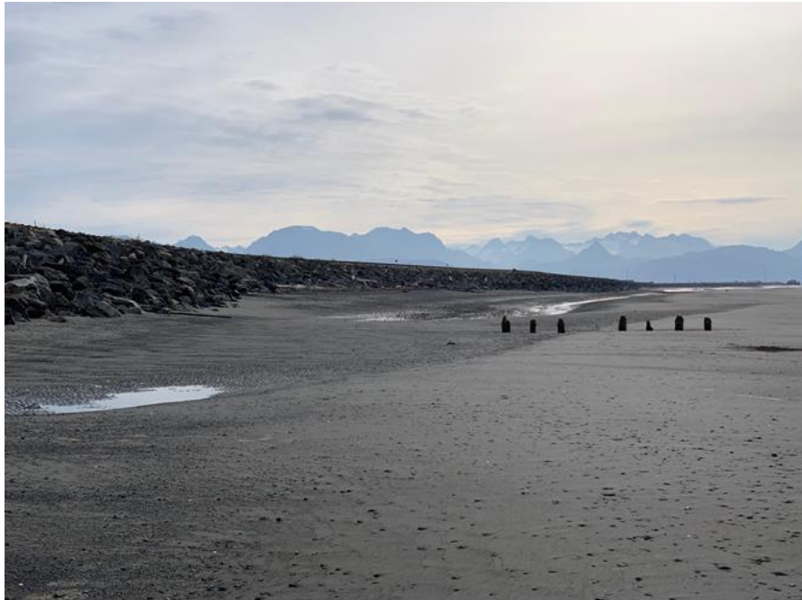
Figure 4. Transition of USACE and DOT&PF revetment projects.
