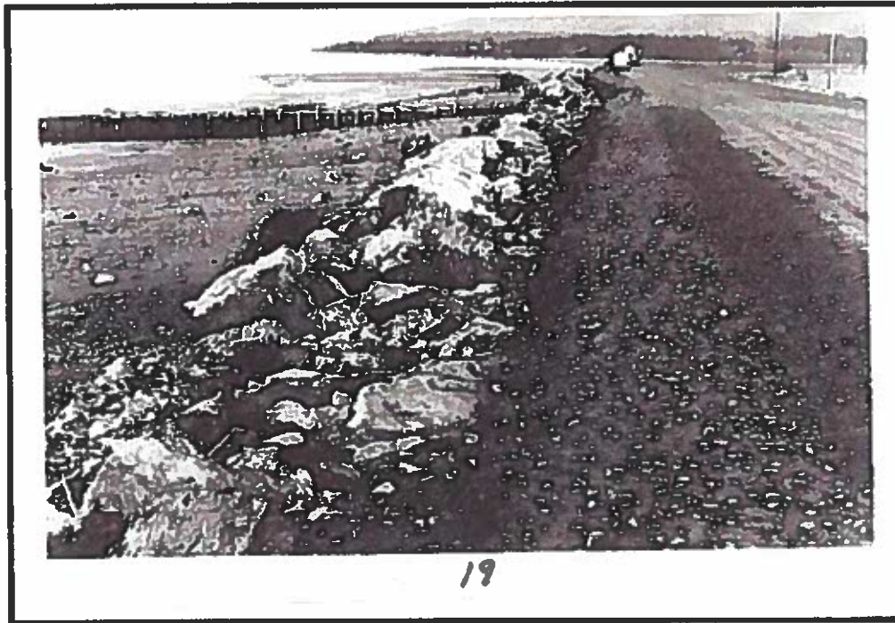
Figure 8. Photograph taken in 1966 of the rock riprap placed along the shoreline in proximity to Groin No. 1, Homer Spit, AK. (Weaver, 1966).
