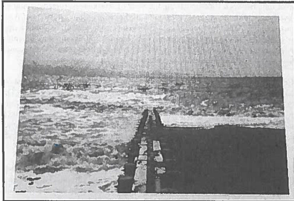
Figure 5. 1963 Photograph of Groyne No. 4 taken in 1963, illustrating the destructive type of wave action along the down drift side, Homer Spit, AK. (Stanley and Grey, 1963).
