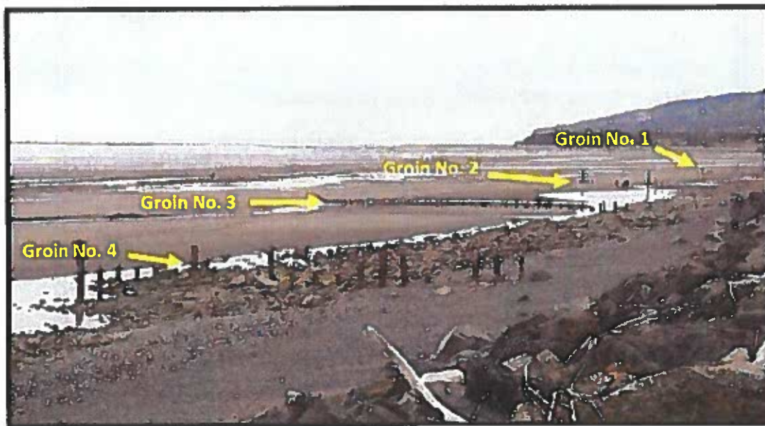
Figure 9. Photograph taken in 2012 of historically constructed wooden timber groins on Homer Spit, AK.
