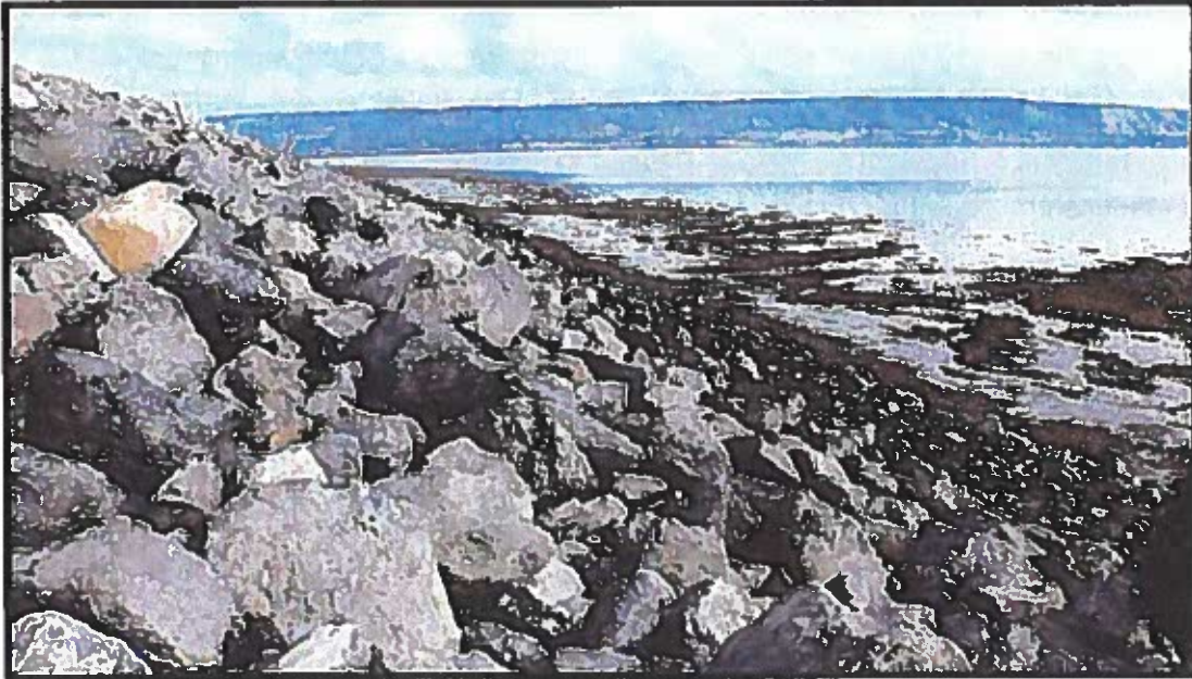
Figure 59. Armor stone riprap protecting the shoreline at the New Harbor Staging Area disposal site, Homer Spit, AK.
