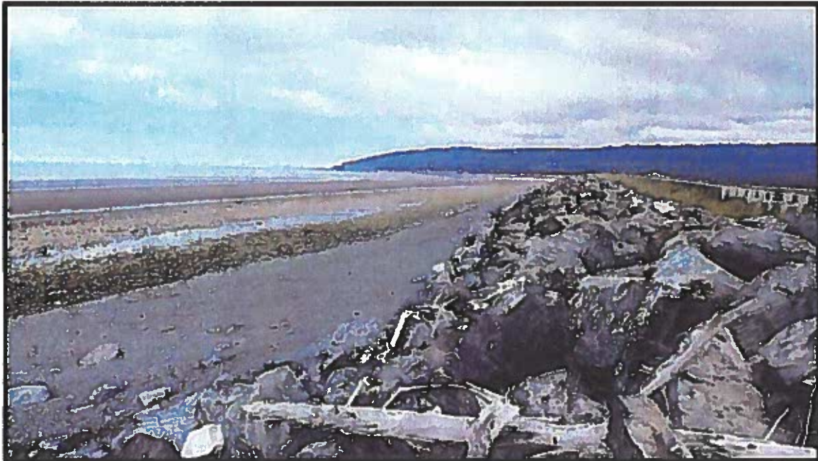
Figure 20. Homer Spit beach nourishment area BN 2, view to northwest, illustrating the rock revetment and offshore topography. Note transition from toe of revetment to gravel beach to band of cobble/tide pools to sand/mud flats.
