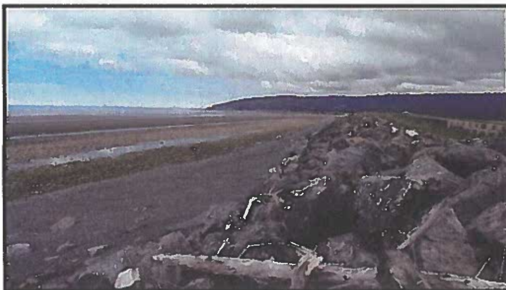
Figure 14. BN 2 physical setting adjacent to rock revetment protecting Homer Spit Road.
