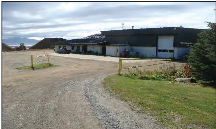
The City of Homer Public Works department’s equipment and fleet and personnel have outgrown the current facility, which is also located in a tsunami inundation zone.
