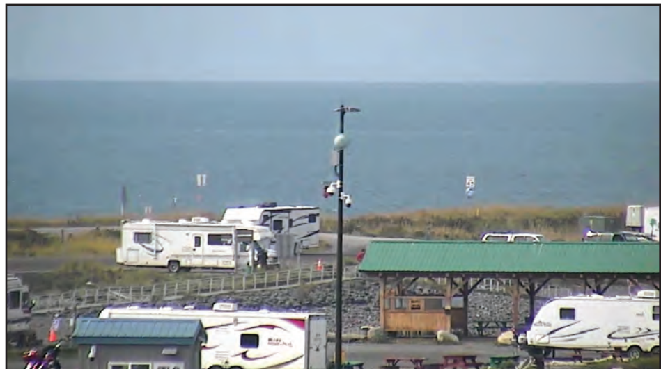
Security cameras, pictured here, center, allow harbor officers to gain situational awareness before responding to an event, to verify details of recorded events and monitor progress of evacuations or check on inundation during tsunami events.
