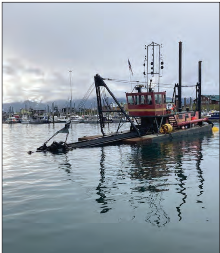
A dredge in Homer Harbor during the US Corps of Engineer’s annual dredging of the harbor’s navigable channel.
