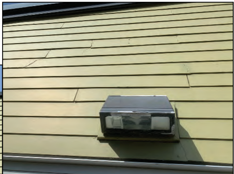
Examples of damaged and broken siding on the library's south-facing wall (at left) and above the library's back door (at top).
