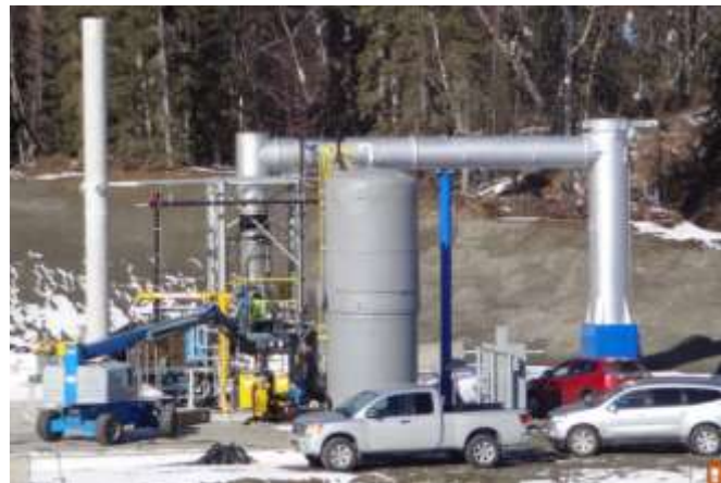
Figure 51. Installing Leachate Evaporation System, Central Peninsula Landfill
