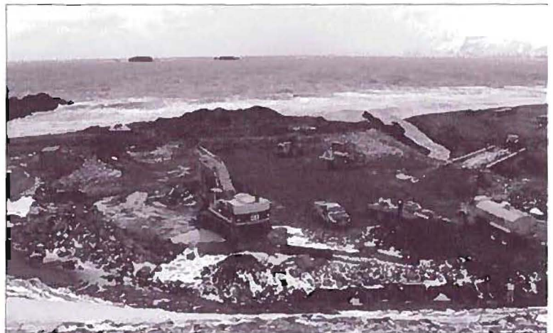
Akutan Airport, Kiewit Infrastructure West
