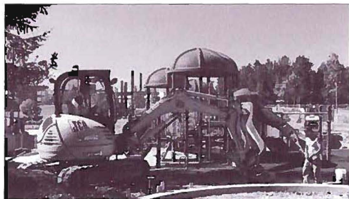
Cuddy Park Playground, Anchorage, JTA Construction
