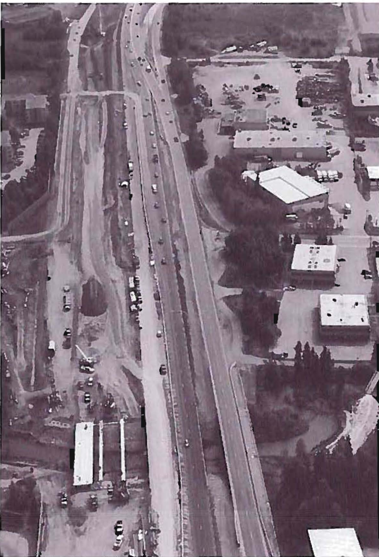
Seward Highway Reconstruction, Anchorage, QAP
