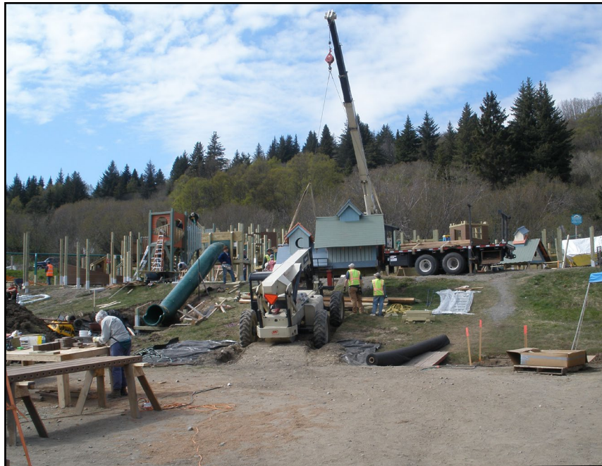
Karen Hornaday Park was a construction site for one week during the Summer of 2012 when the community came together to build a state of the art playground.
