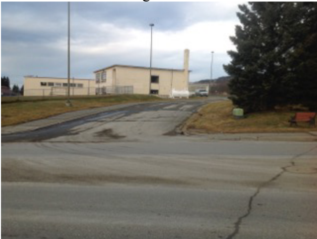
and the HERC building
