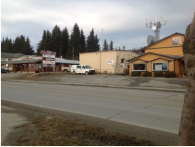
Across the street, two nice looking buildings with a large shed in need of painting between them. Could plant more vegetation around signs. Could add large planter on lot line between ACS and Upstairs Boutique building to break up this long stretch of concrete.
