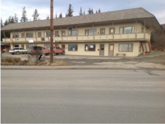
Rough broken pavement:
