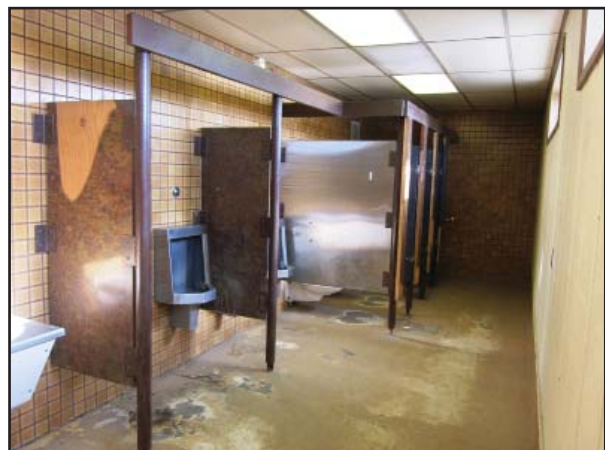
Ramp 2 Restroom, at forty-three years old, needs upgrading for sanitation, energy efficiency and maintenance cost reduction..
