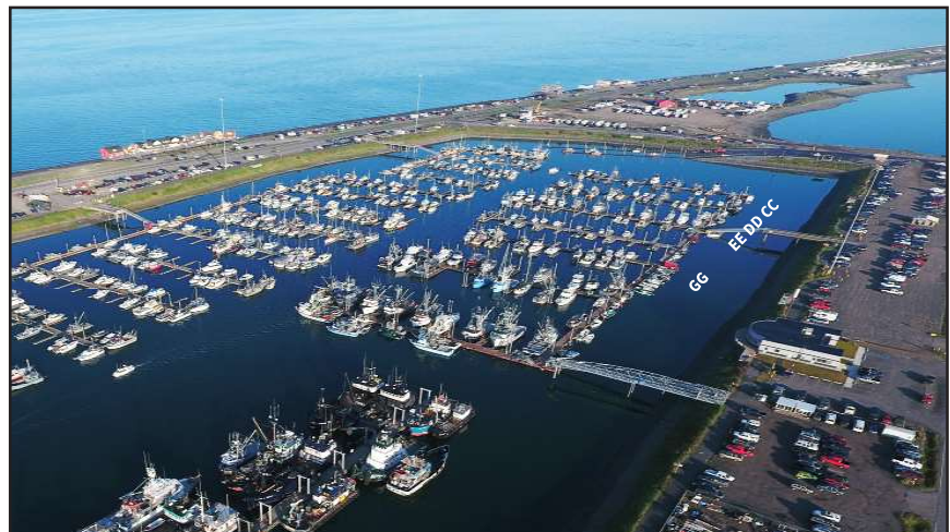
System 4 ramps to be replaced next.
