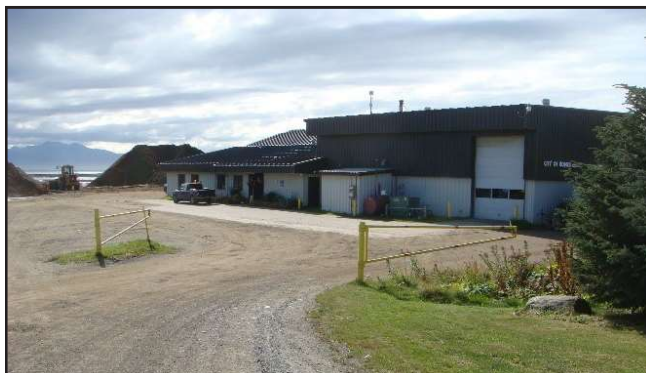
City of Homer existing Public Works facility.
