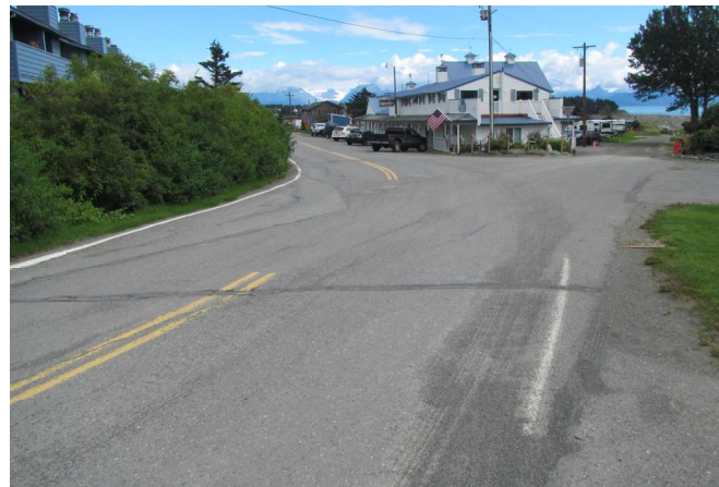
Figure 3- Ohlson Lane at Bunnell Avenue
