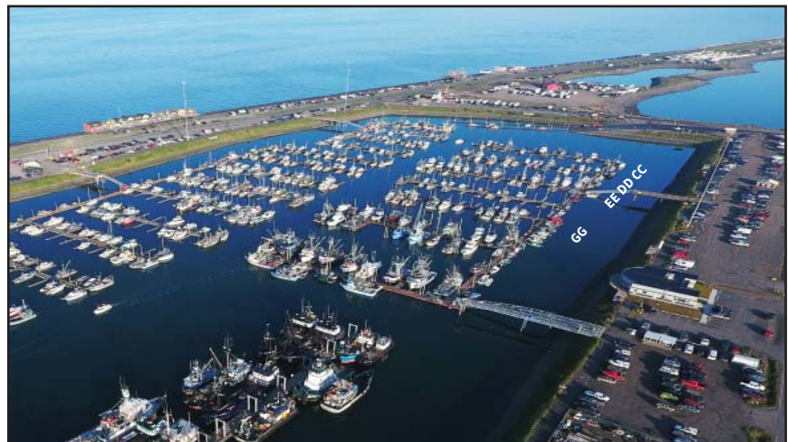
System 4 ramps to be replaced next.
